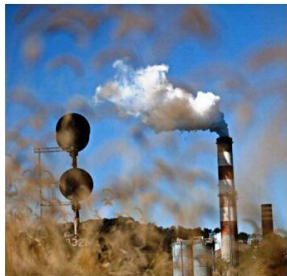
The Mitchell Power Station, a coal-fired power plant built along the Monongahela River in New Castle, Pennsylvania, was shut down last year. Through its Clean Power Plan, the U.S. EPA and the Obama administration have been taking major steps to get coal-fired power plants into compliance with carbon regulations. Credit: Jeff Swensen/Getty Images
